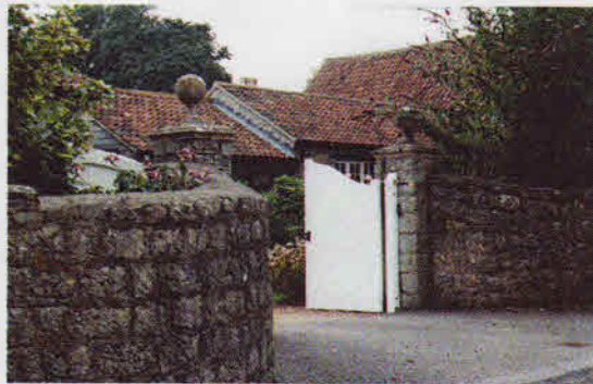
Gate piers - coursed stone wall with cemented top
