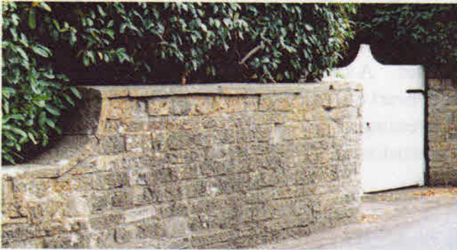
Stone wall with flat coping
