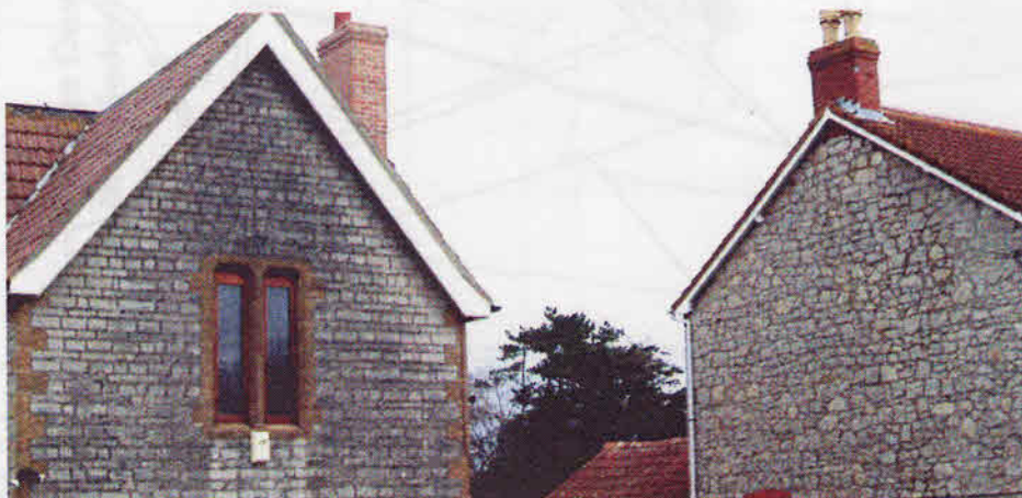
Coursed and surface dressed
